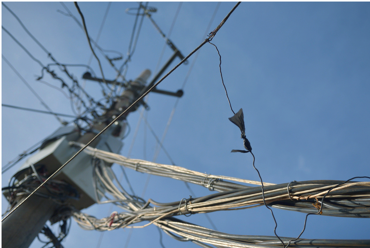
A wire denoted by a piece of polythene tied around it is used to make an illegal connection.
